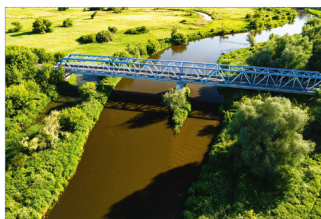
↳ STEEL BRIDGE OVER THE PILICA RIVER ↳ photo: Adobe Stock
