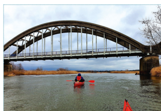
→ BRIDGE IN BIAŁOBRZEGI → photo: Piotr Dylewski
