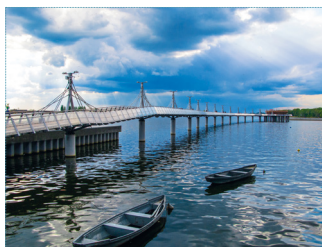
→ PIER IN PŁOCK → photo: Adobe Stock
