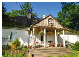
↑ MANOR HOUSE IN GŁUCHY ↑ photo: GHG
