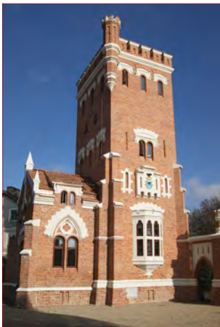
↑ WATER TOWER HOUSING THE KRASIŃSKI FAMILY MUSEUM ↑ photo: arch. UG w Krasnem
