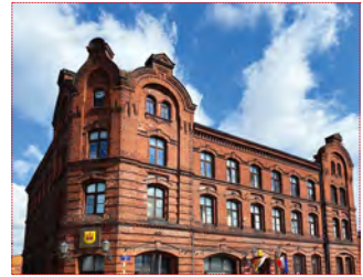
HISTORIC TOWN HALL photo: arch. MROT
