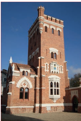
↑ WATER TOWER HOUSING THE KRASIEŃSKI FAMILY MUSEUM ↑ photo: arch. UG w Krasnem
