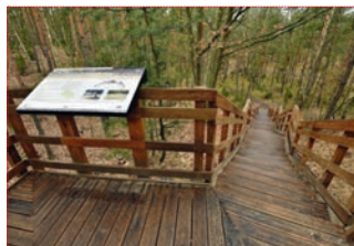
FOOTBRIDGE ON ŁUZOWA HILL photo: arch. Kampinoski, PN
