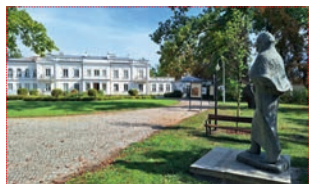
HEADQUARTERS – SANNIKI PALACE photo: ECA Archive
