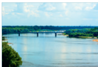
→ STEEL BRIDGE OVER THE VISTULA IN NOWY DWÓR → photo: Grzegorz Hubert Gerek
