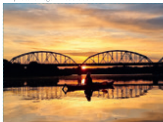
→ BRIDGE IN NOWY DWÓR → photo: Piotr Dylewski
