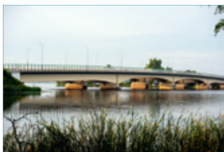
→ ROAD BRIDGE IN ZEGRZE → photo: Grzegorz Hubert Gerek
