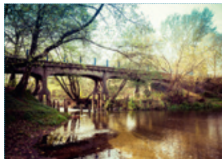
→ NARROW-GAUGE RAILWAY BRIDGE IN OTWOCK → photo: Adobe Stock
