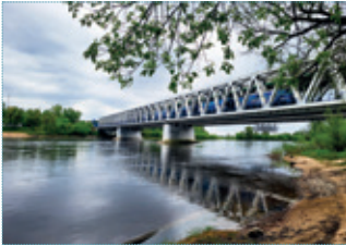
↳ BRIDGE OVER THE NAREW RIVER IN MODLIN ↳ photo: Marcin Oporski
