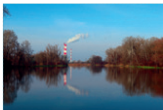
→ SIEKIERKI COMBINED HEAT AND POWER PLANT → photo: Adobe Stock
